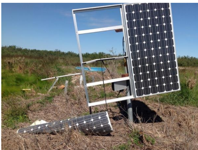
Figure 1. Solar panel damage at a freshwater pond following Hurricane Harvey, August 2017. Note storm surge wrack line in foreground.
